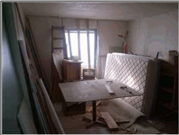
Room 190 - Under renovation.jpg
