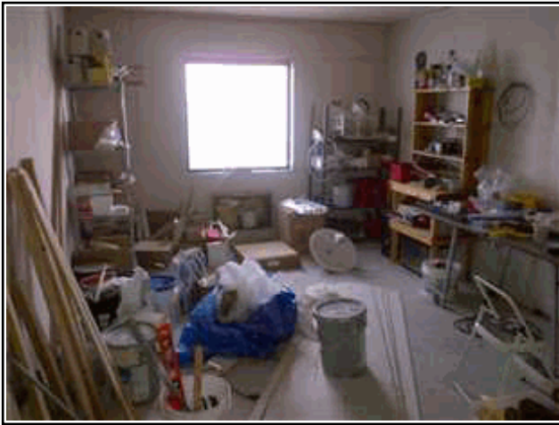
Room 191 - Under renovation.jpg
