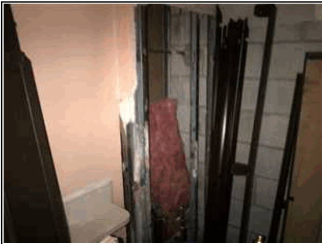
Room 188 - Under renovation B.jpg
