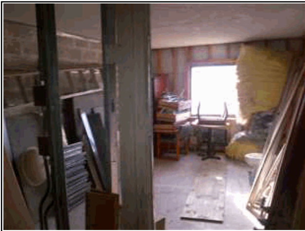
Room 192 - Under renovation.jpg
